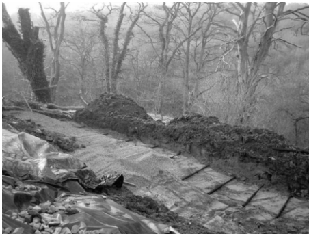
Figure 5. Laying out of the perforated drainage pipes and the filter layer.
