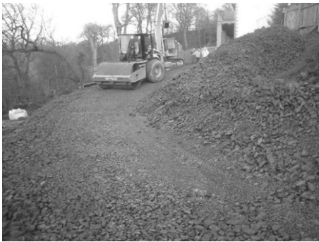
Figure 6. Compaction of the rockfill in layers.
