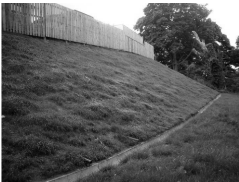
Figure 7. Completed vegetated slope with contour channel drain at the toe.
