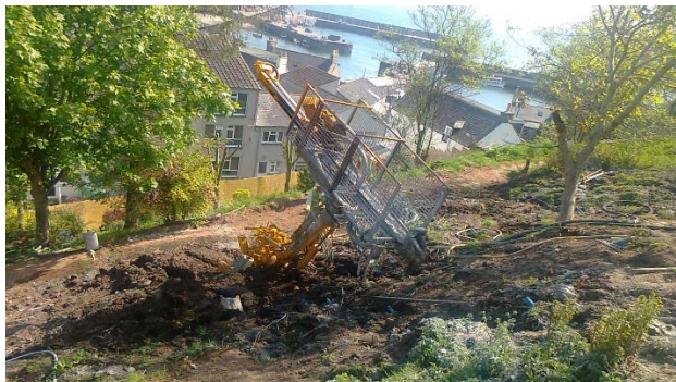
Figure 3 Soil nailing rig positioned on site. A short section of soil nail can be seen on the slope in front of the rig.
