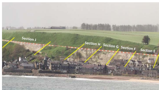
Figure 1. Site area with delineated soil nailing sections
