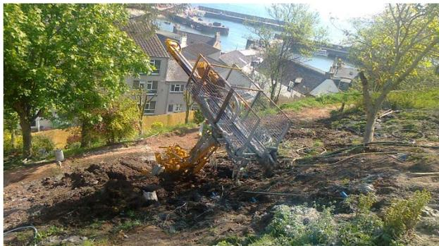
Figure 3 Soil nailing rig positioned on site. A short section of soil nail can be seen on the slope in front of the rig.
