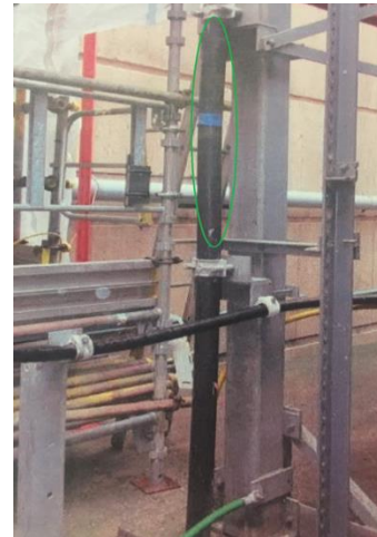
Figure 3. 275kV OF cable (Blue Phase) – the area marked in the green ellipse was observed to have a 5.2°C temperature rise.
