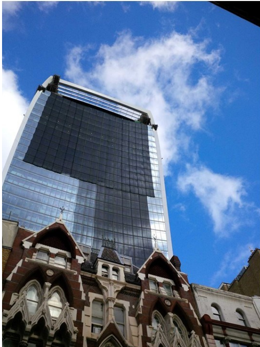
Figure 5. 20 Fenchurch Street – a) looking towards the South Façade from Eastcheap showing temporary covering and b) schematic showing angle and focus of solar beam for early September
