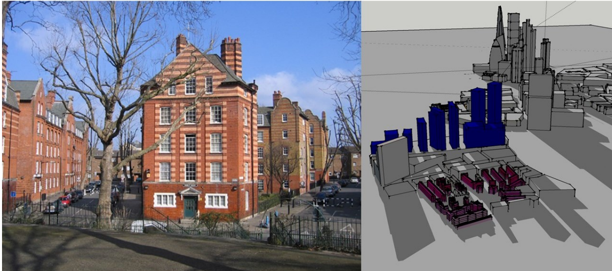
Figure 7. a) The Boundary Estate showing current levels of solar access into streets b) Bishops Goods Yard showing and 3D model of the proposed, but now in abeyance, Bishopsgate Goods Yard Development overshadowing the underlying Boundary Estate – both images are for February early afternoon.
